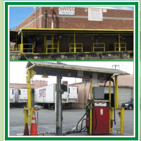
Previous Swiss Dairy factory
