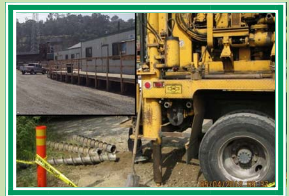
Augers being removed after drilling at Humboldt Site
