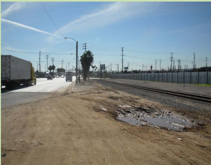
Alameda Street Before Widening.
