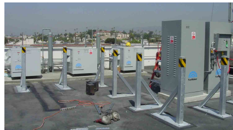
3 Multi-Compressor Units and 1 Fast Fill Unit at the Hollywood Yard
