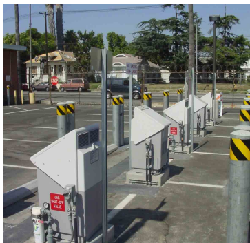
Row of 5 FuelMaker Single Compressor Units at the South Los Angeles Yard
