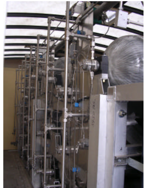
Inside the hydrogen fueling station located at Beaudry and Second Streets near downtown Los Angeles. Hydrogen gas is stored in a series of twenty tanks at increasingly higher pressures.
